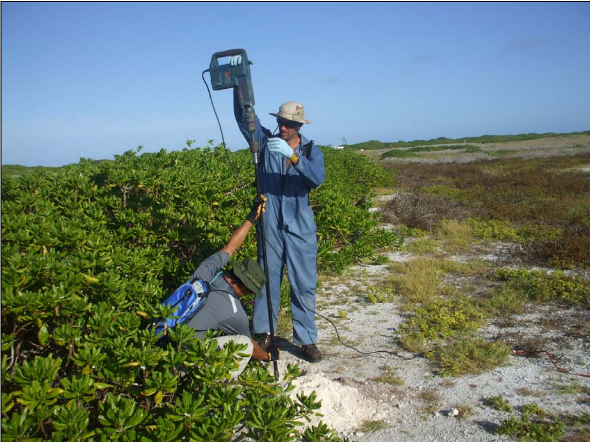
Installation of Solinst Drive-point piezometer using Bosch Roto-Hammer.
