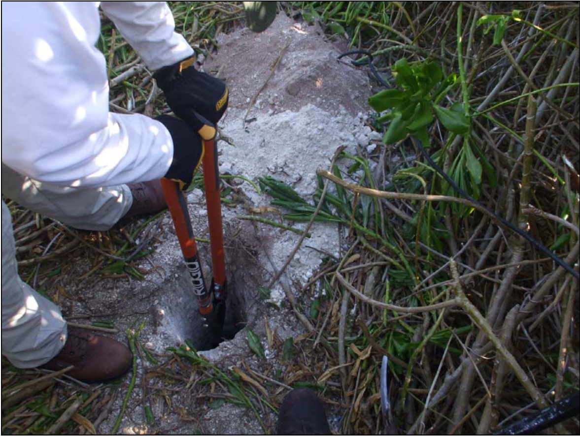
Pre-digging of piezometer location.
