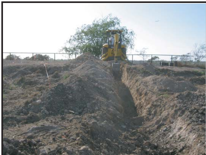
Photo 9: Typical view of trench excavation
