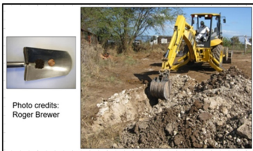
Figure 2-2. Subsample sizes and representation. A single arbitrary clump of soil will not have the same concentration, and therefore properly represent, the volume of soil being excavated.
